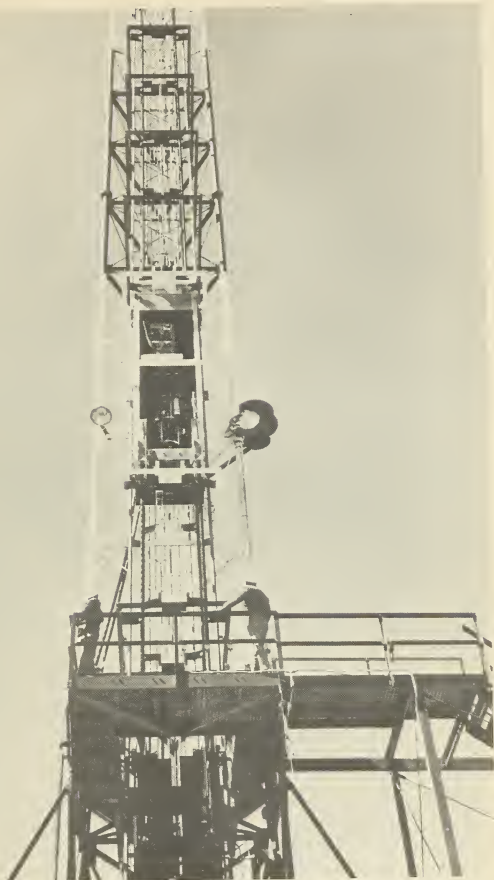
Fig. 8 The Health Physics Research Reactor mounted on hoist car on the BREN tower.
